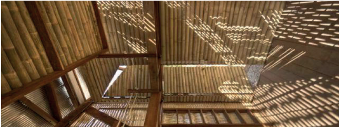
Rural Thai Building in Tak, South East Asia – design by TYIN tegnestue Architects
